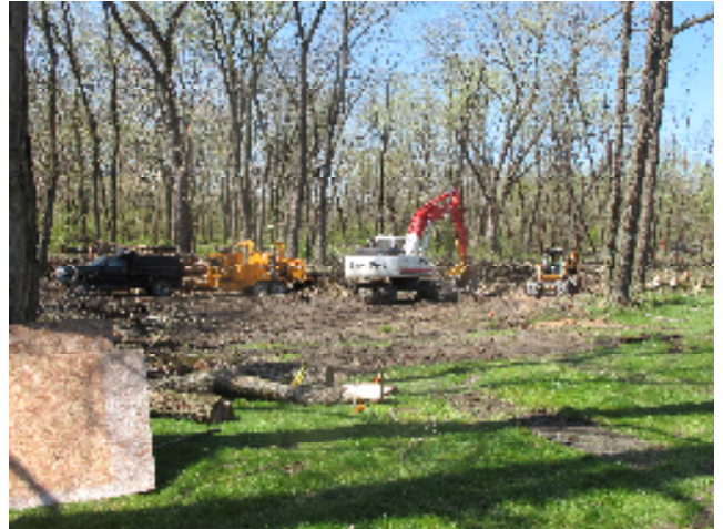
Heavy equipment begins the parking area project
