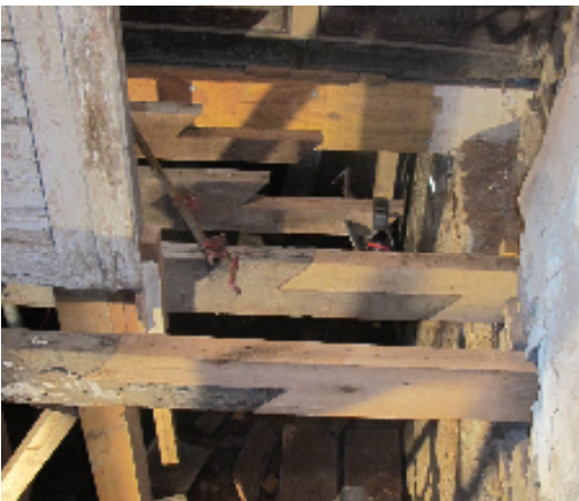
Scarf-jointed floor joists at Douglass House
