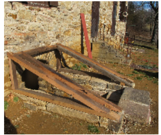
Cellar cap frame at Keim House
