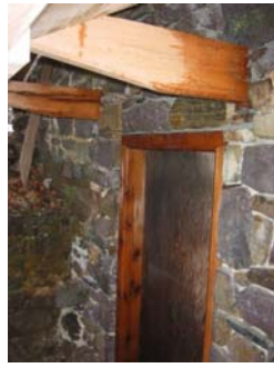
Replacement oak hood outlookers over restored kitchen doorway jambs and lintel
