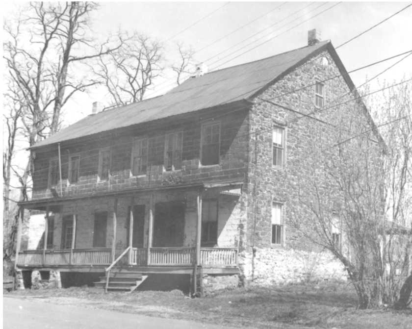
White Horse Inn pre-restoration 1971. Notice the three chimneys, the Victorian era porch and the double entry doors. See this image and many more by visiting the online archive. A link to the archive can be found on the Trust's website www.historicpreservationtrust.org
